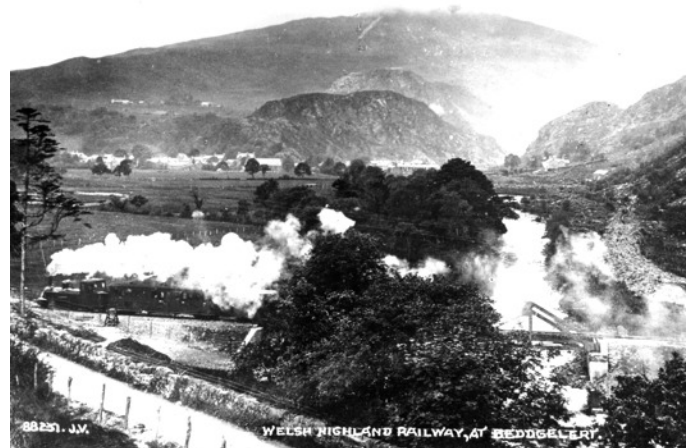
Moel Tryfan heads a short train across the bridge at Bryn-y-felin en-route to Beddgelert. The earlier PBSSR works are visible up the right-hand side of the image. Valentine 88231.JV - Arch 0235
