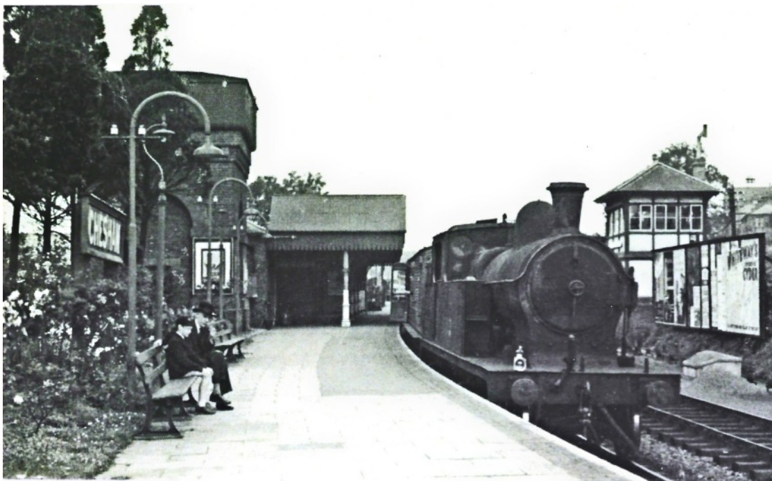
Alfred Croughton shares a station bench with a young Richard Casserley, son of Alfred's contemporary Henry Cyril Casserley. The elder Casserley and Emily Turton, Croughton's wife, were cousins. This photograph was taken by Henry Casserley showing Alfred and Richard apparently indifferent to the locomotive in front of them. That loco was ex-G.C.R. Robinson-designed class 9K 4-4-2T number 193, which by the time this photograph was taken had become L.N.E.R. number 5193. There is a peripheral link to the W.H.R. here as this locomotive was built at the Vulcan Foundry for the G.C.R. works at Gorton, Manchester. When this photo was taken, the loco was shedded at Neasden. - Chesham Station, northwest London - 1946. Reproduced here by courtesy of Mary Casserley.
