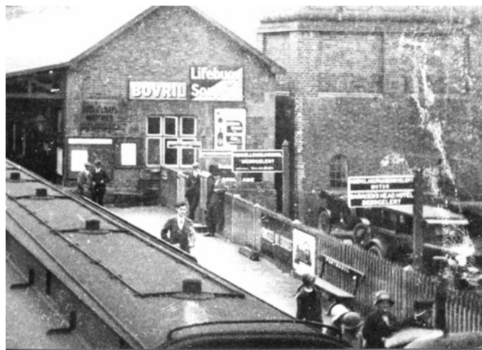
Portmadoc Standard Gauge station in 1926, showing the pick-up area adjacent to the platform with sign-posted motor services to Beddgelert and, specifically, to the Saracen's Head - C.L. Mowat - Arch 4934
