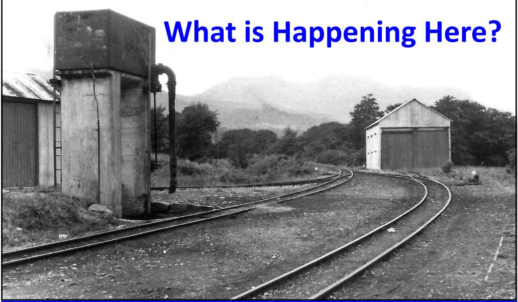
Adjacent to the main line stands a pair of reinforced concrete pillars that between 1923 and 1937 had a water tank on top. They represent one of the few tangible remains of the railway from that period. Beyond is a corrugated iron hut which is a replica of the original 'lamp-room' that adorned the site.
